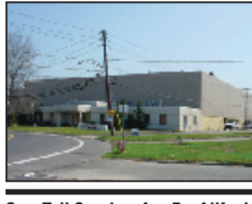
Sam Tell Co. site after Roof lifted to 35' clear
