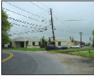
Sam Tell Co. site. Roof 14' clear
