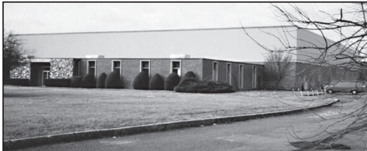
After picture of building after being lifted to a 29 ft. clearance
