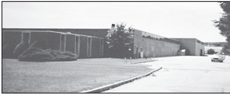
Before picture of a roof with a 16 ft. clearance
