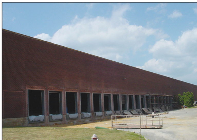
Forsgate property before renovation
