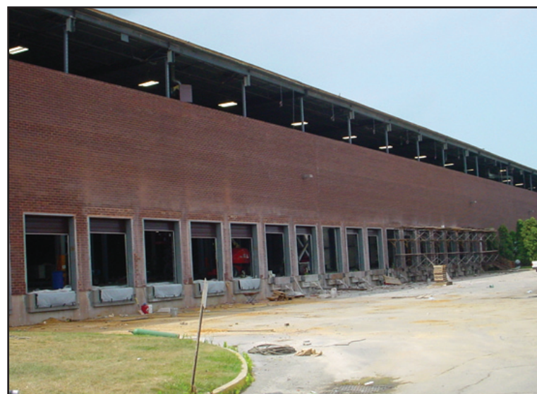
Forsgate property during renovation
