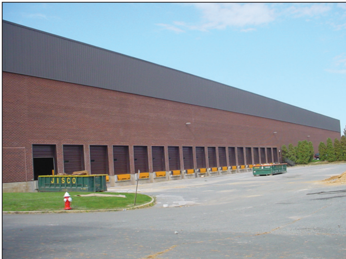
Forsgate property after renovation
